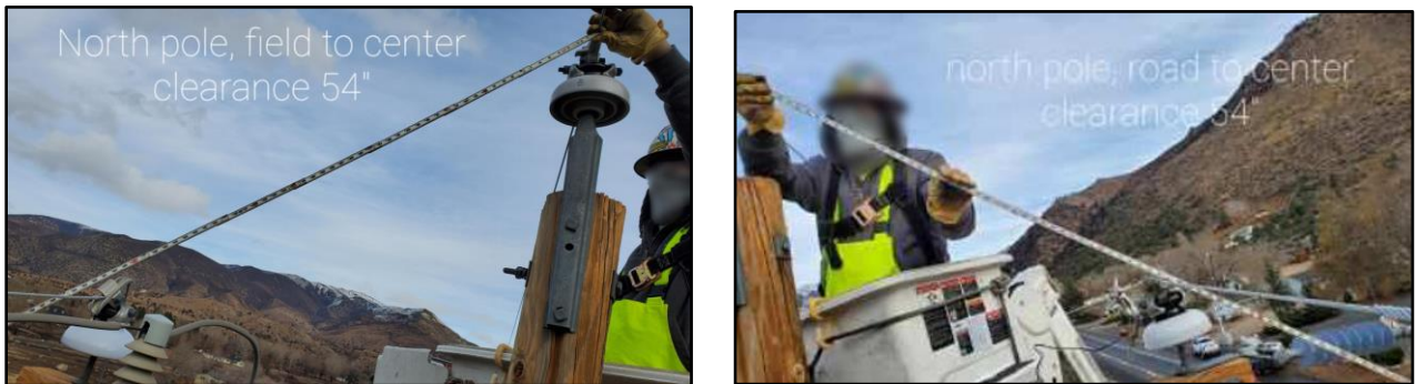
Figure 8: Annotated Demonstration of Measured Radial and Calculated Horizontal and Vertical Conductor Clearances
